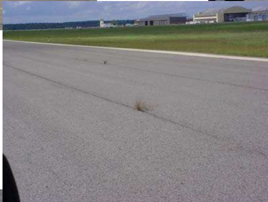
Runway-36 exhibiting signs of grass growing in longitudinal cracks.
