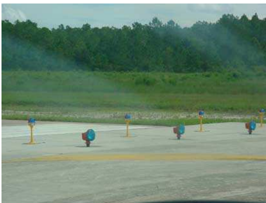
Threshold lights at Runway 36R end.
