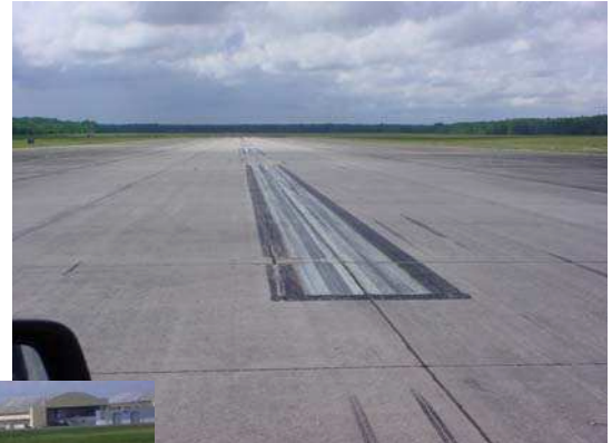
Rubber buildup beginning to obscure runway centerline marking.
