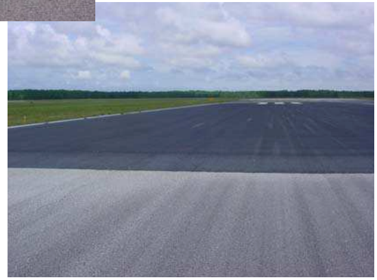
Recent overlay on Runway 18R-36L.
