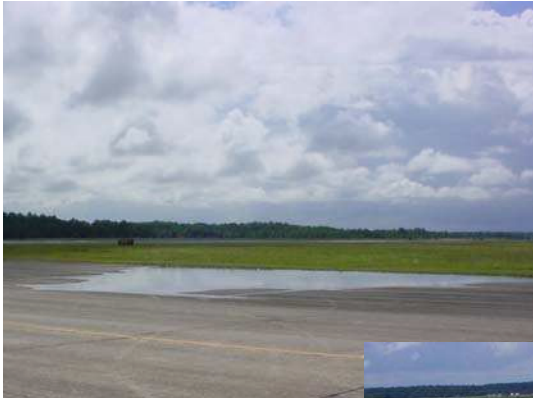
Ponding on Taxiway A-1.
