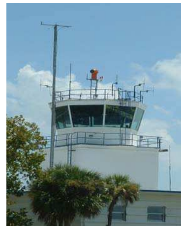
Rotating Beacon (on top of ATCT)
