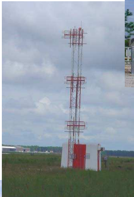
Glide Slope Antenna
