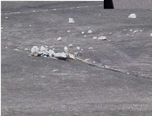
Spalling on Runway 18L-36R.
